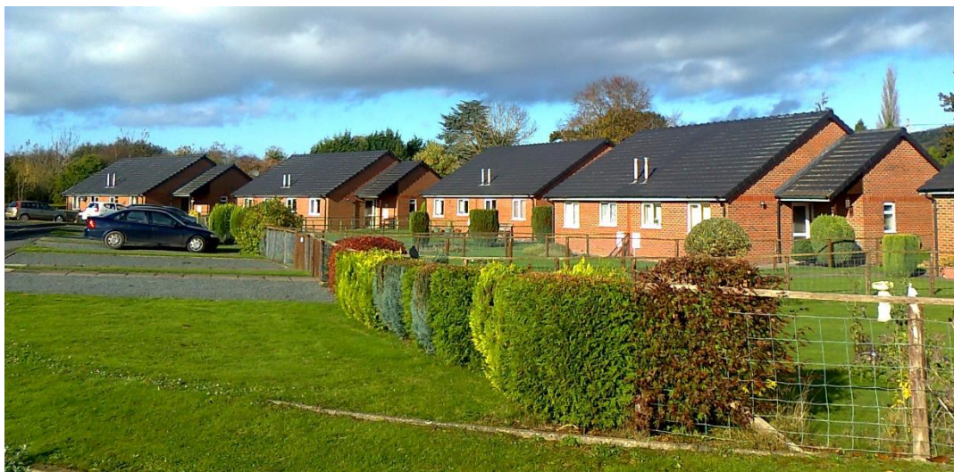
Affordable Housing Scheme, Barnfield
